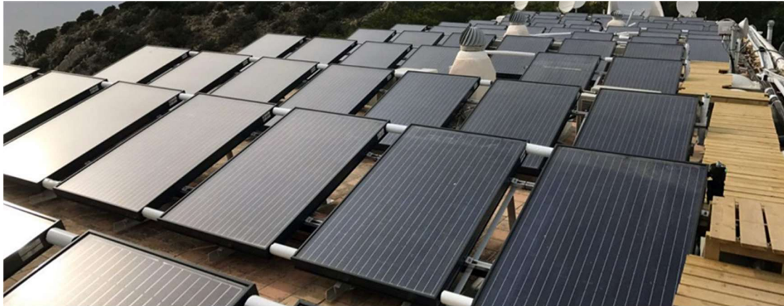
Figure 4: Installation of Ecomesh PVT panels [30]
