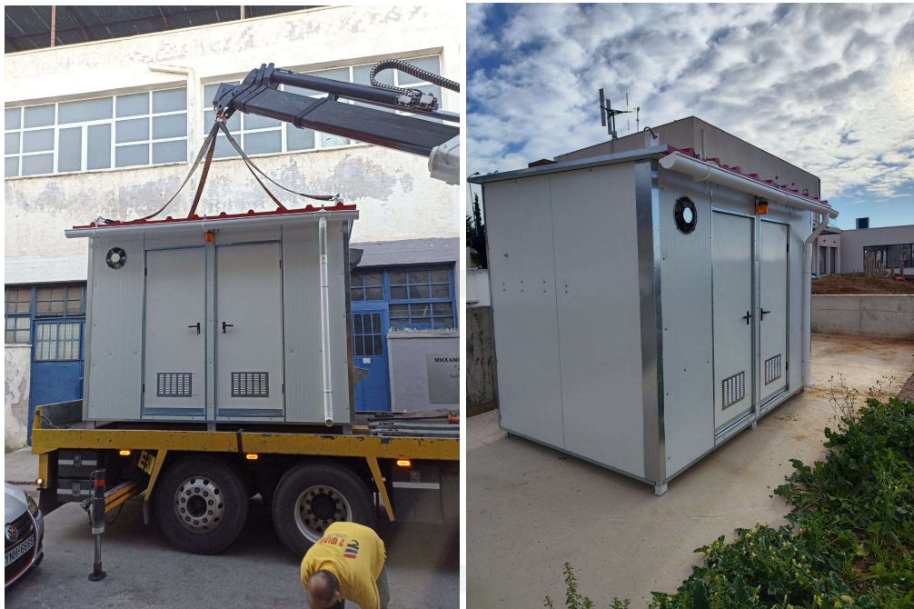
Figure 44. The completed and tested Ministor system leaving premises of Psycrotherm (left) and installed at CERTH (right).
