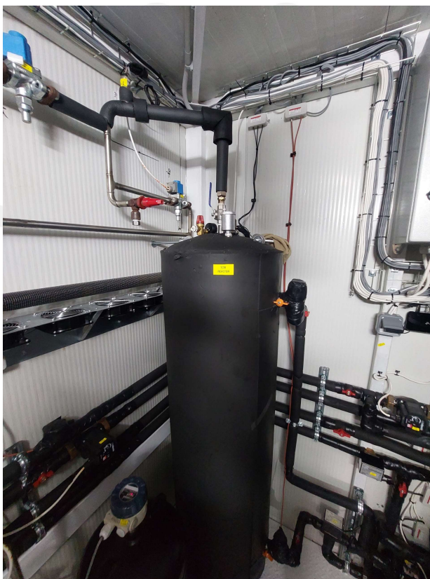
Figure 12. The TCM reactor with the safety valves completed.
