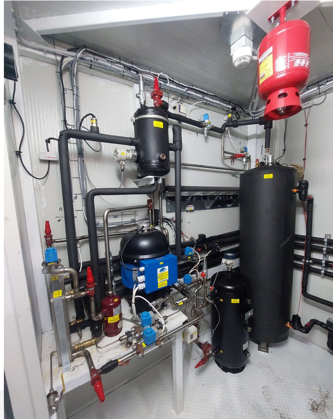
Figure 13. The fully completed MiniStor unit with the integrated TCM reactor.
