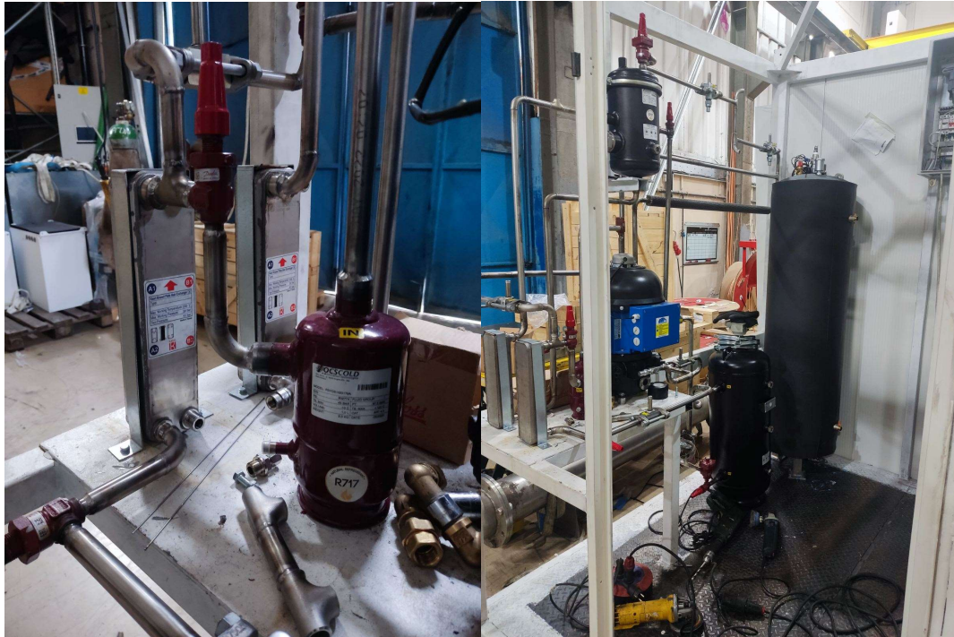
Figure 7. The ammonia circuit during the MiniStor assembly.
