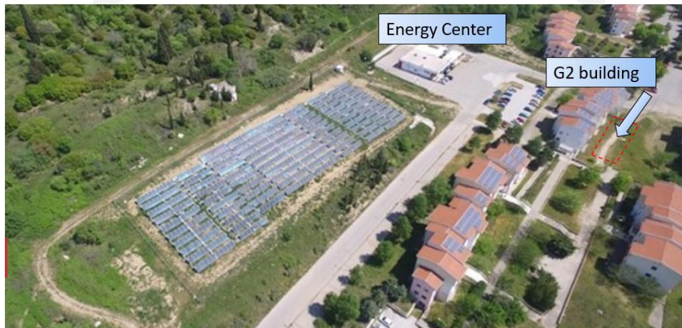
Figure 8: Birdview of the DUTH's demo site location for the MiniStor system.
