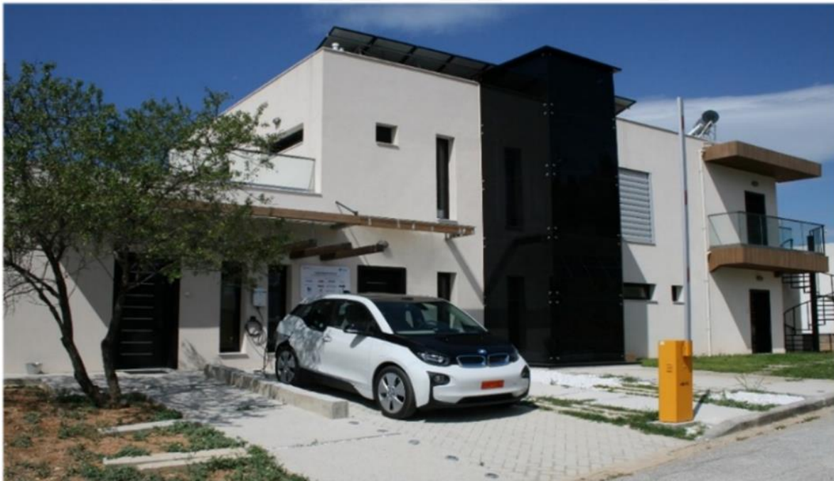
Figure 20: Picture of the demonstration site in Thessaloniki.
