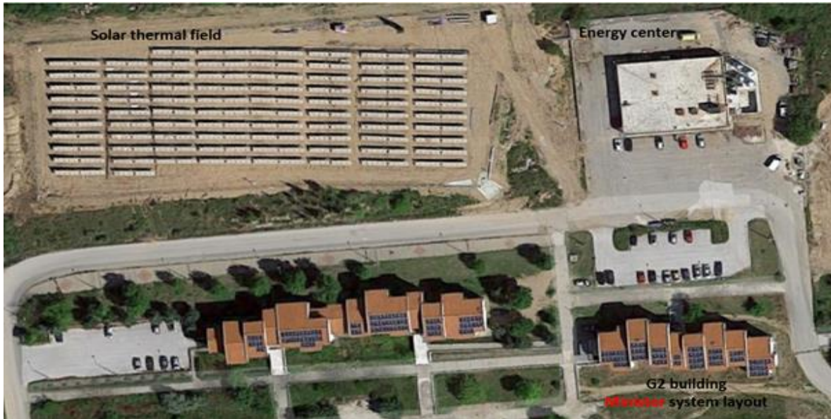
Figure 8: Satellite image of demonstration site in Kimmeria.
