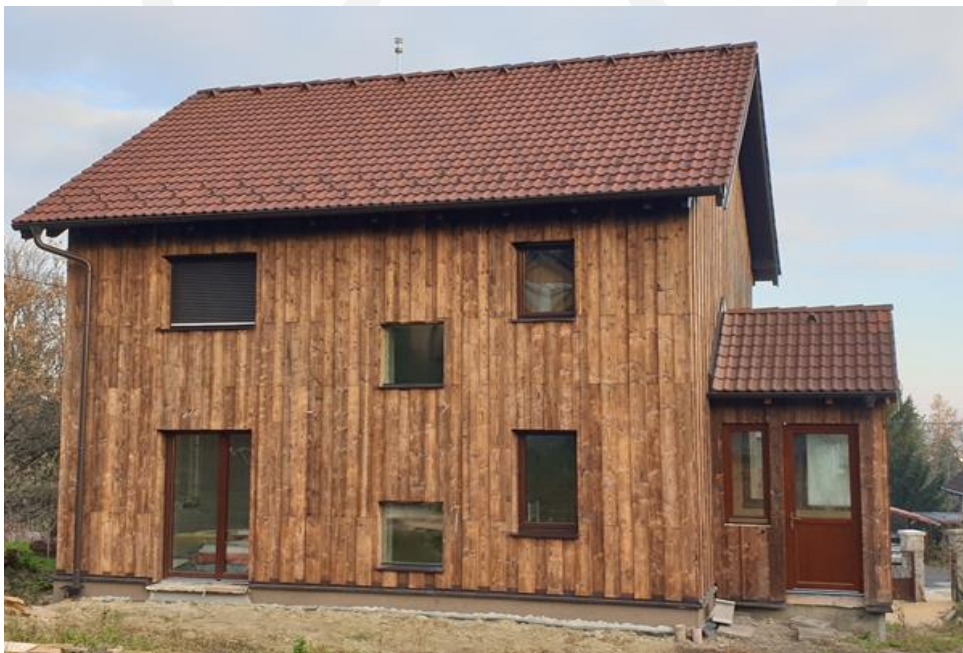
Figure 16: Picture of the demonstration site in Sopron.
