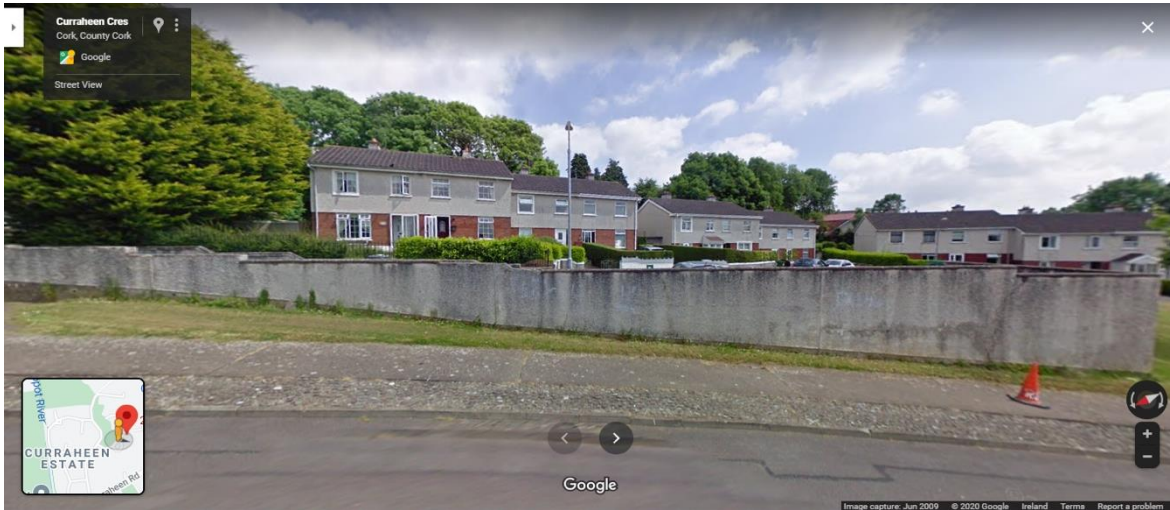
Figure 4: Google Streetview image on the demonstration site (end house on the left).
