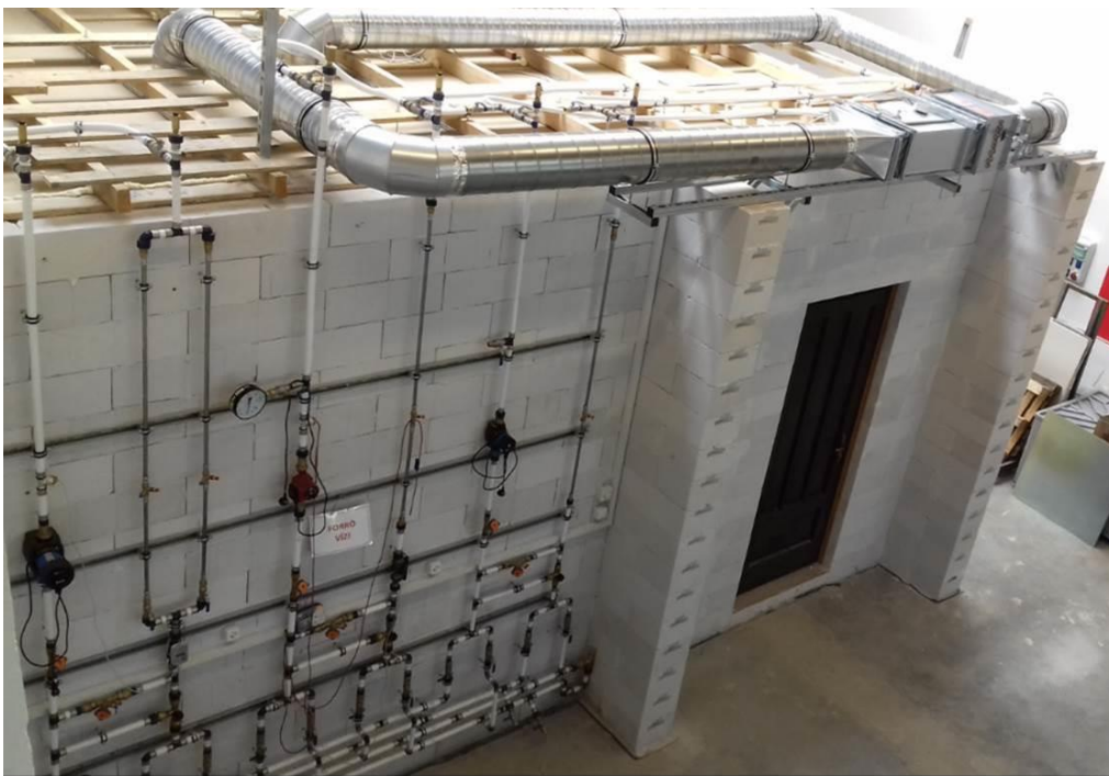
Figure 6-Hydraulic connection of the testing facility (EMI labs Sopron Hungary). Source: EMI
